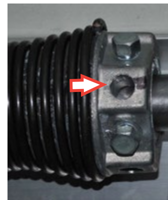
Spring winding plug holes
