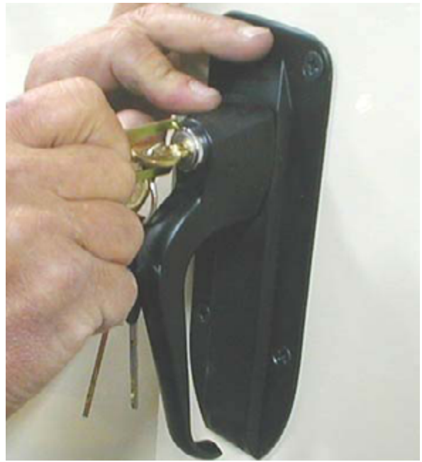
Remove and reuse the existing lockset
